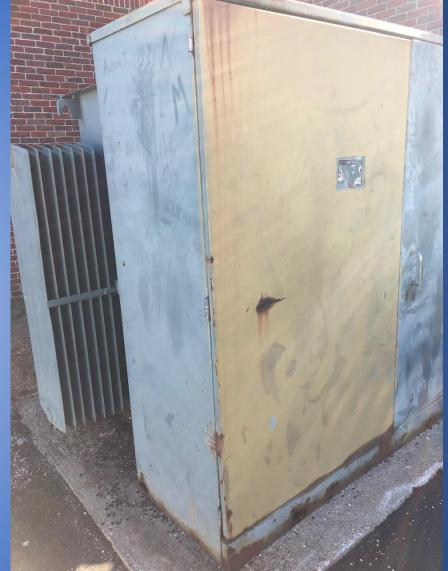
MUES -Switchgear Replacement \$100,000 Installed in 1992. Life expectancy exceeded
