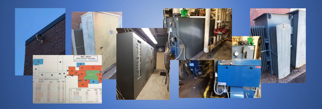
MHS-Transformer Replacement \$75,000 Installed in 1977. Life expectancy exceeded.
